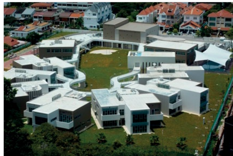
Aerial view of SAAC at Elliot Road.
